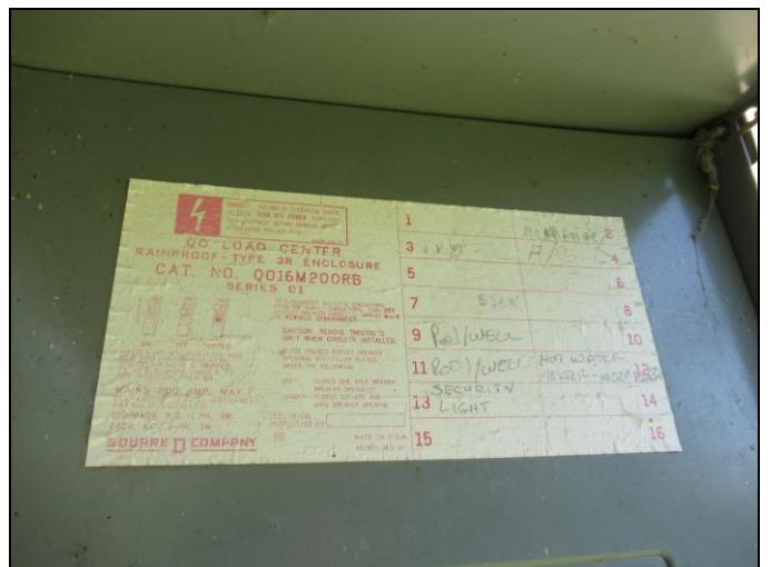
Subject Main Distribution Panel Interior Door Label
