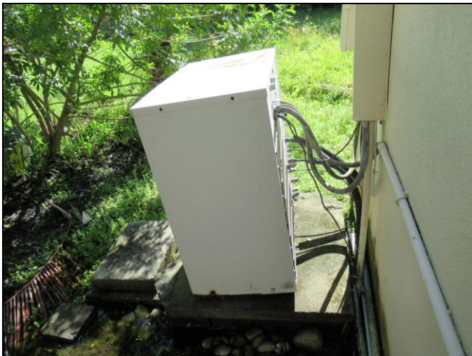
Subject Air Conditioning System
