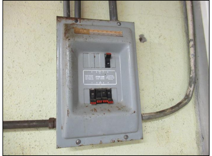
Subject Secondary Distribution Panel Interior Door Label
