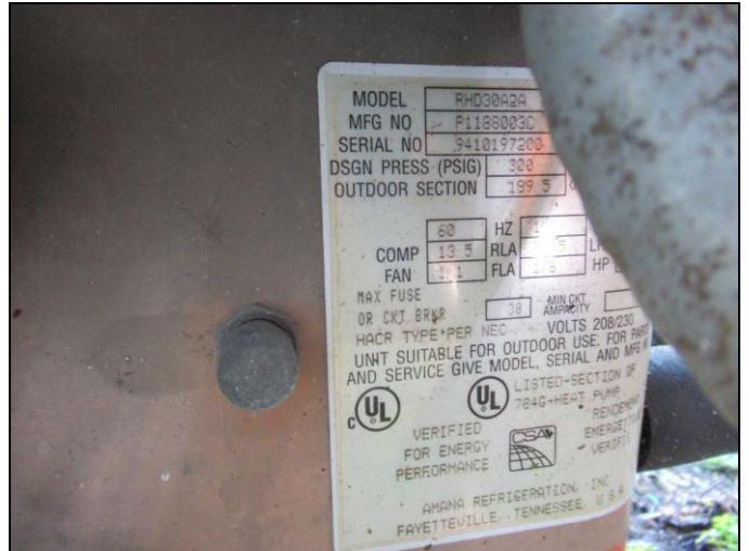
Subject Air Conditioning System Data Tag
